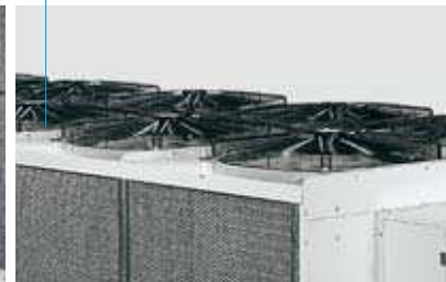
Axial fans with various rotational speeds
