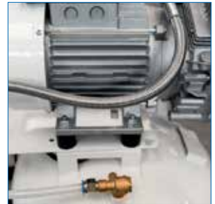
Pump unit mounted on anti-vibration devices
